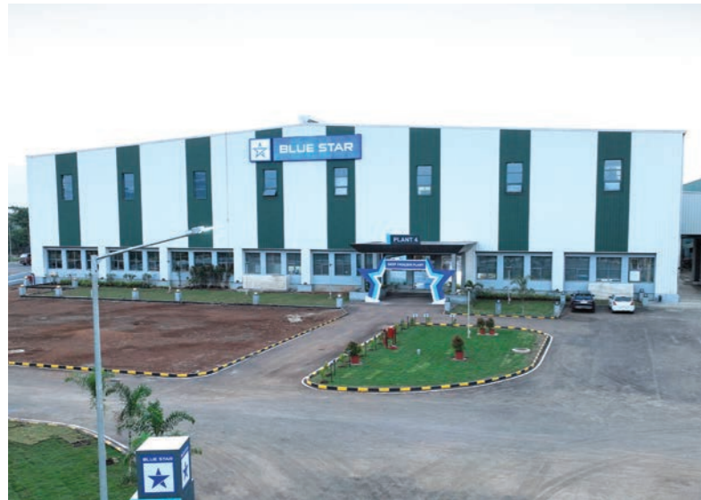
Wada – Deep Freezer Plant
